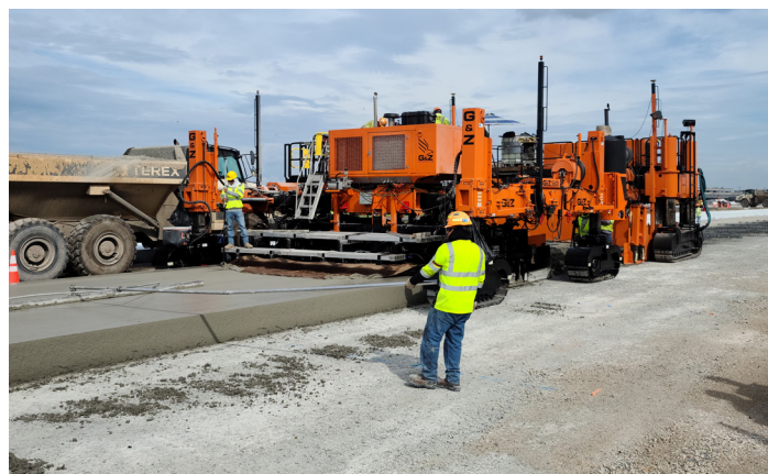
Taxiway Reconstruction Joint Base Andrews, Maryland 2021
