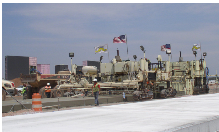
K & K7 Taxiway Rehabilitation Washington Dulles International Airport (IAD) 2007
