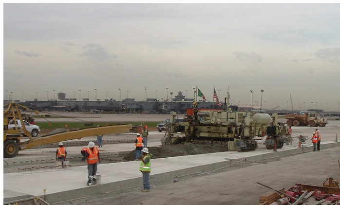
KK2 & K3 Taxiway Reconstruction Washington Dulles International Airport (IAD) 2005
