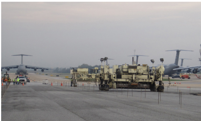
Taxiway Reconstruction Dover Airforce Base, Delaware 2011
