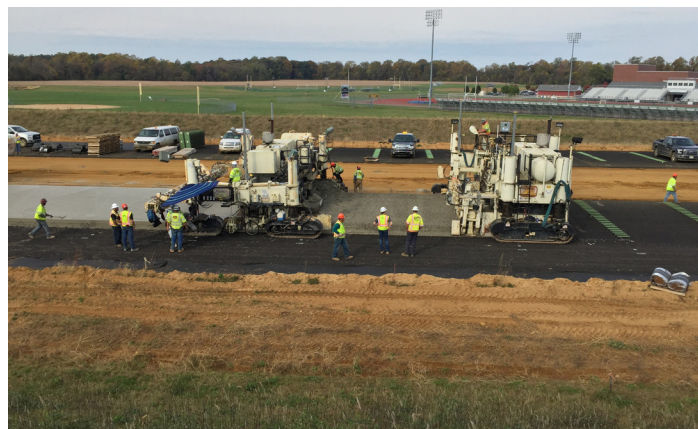
Highway Construction U.S. Route 301, Delaware 2008
